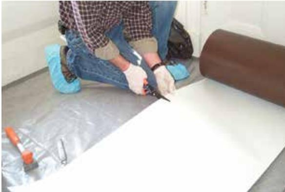
Dry fit to determine if edge cuts are necessary.
