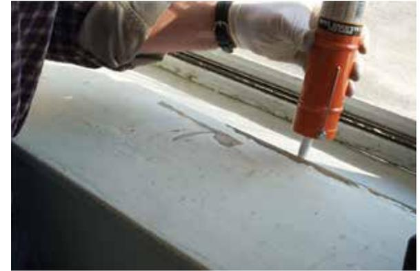
**Apply caulking to window well only, not directly on coil stock.**
