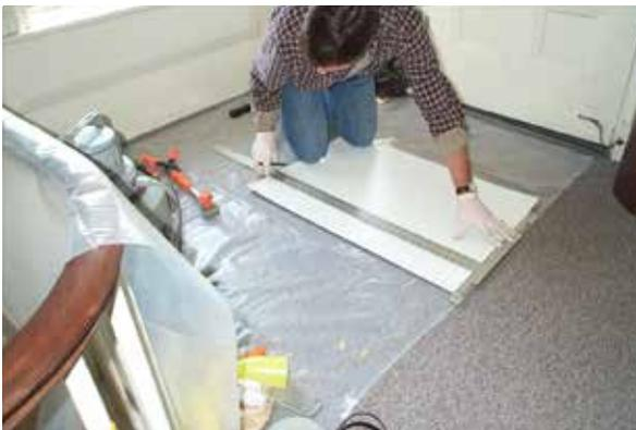
Cut edges to fit shape of jamb.
