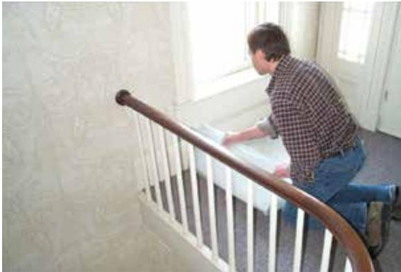
Check area for any remaining dust or debris and HEPA-vacuum or wipe if necessary.
