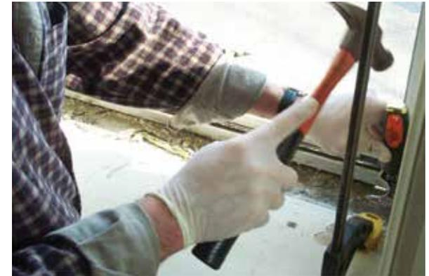
**Wet-scrape deteriorated paint from window well.**
