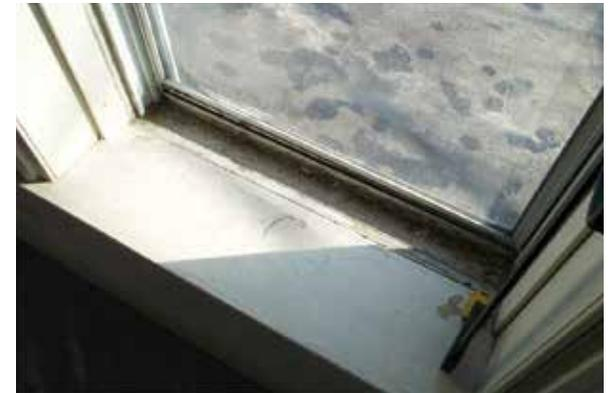
**HEPA-vacuum loose debris from window well.**
