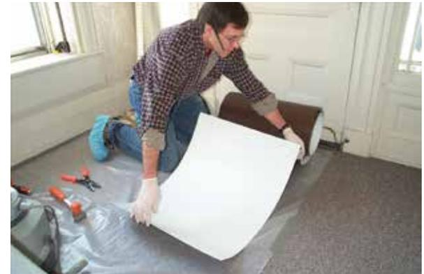
Coil stock may also be cut using tin snips.
