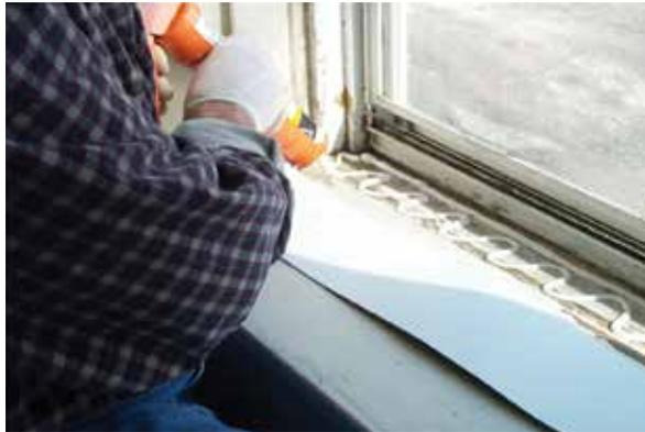
**If caulking lower edge, leave weep holes for water to escape.**
