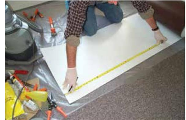
**Coil stock may be cut by scoring with a utility knife, using a straight edge as a guide.**
