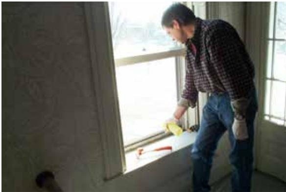
**If possible, create a gap under window parting bead to allow coil stock to be slid underneath.**
