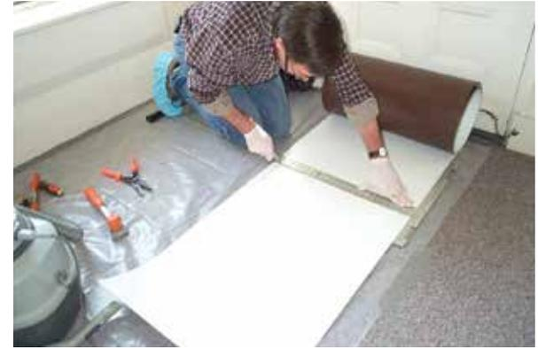
**Bend coil stock as shown to break on a scored line.**
