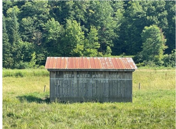
High water mark from the 2023 flood on Route 14 between Morrisville and Hardwick
