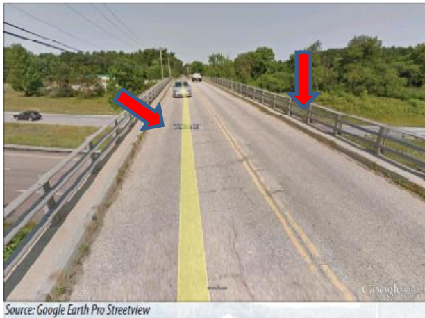
Figure 6: West Milton Bridge
